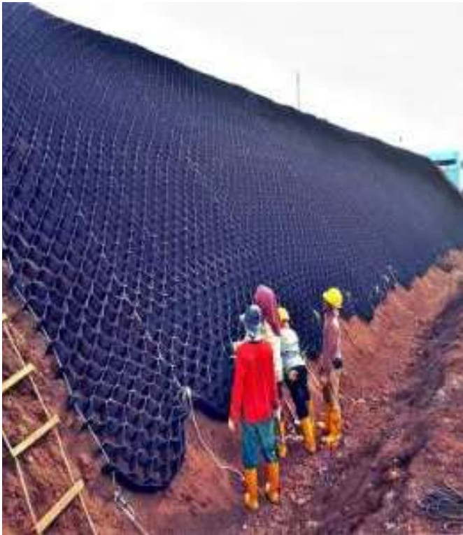
Slope Protection with Geo Cell
