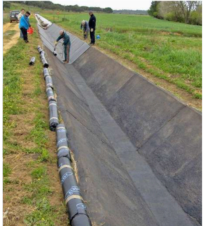
Canal Lining Work
