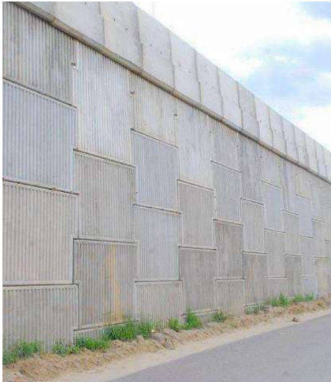
RE wall with Panels
