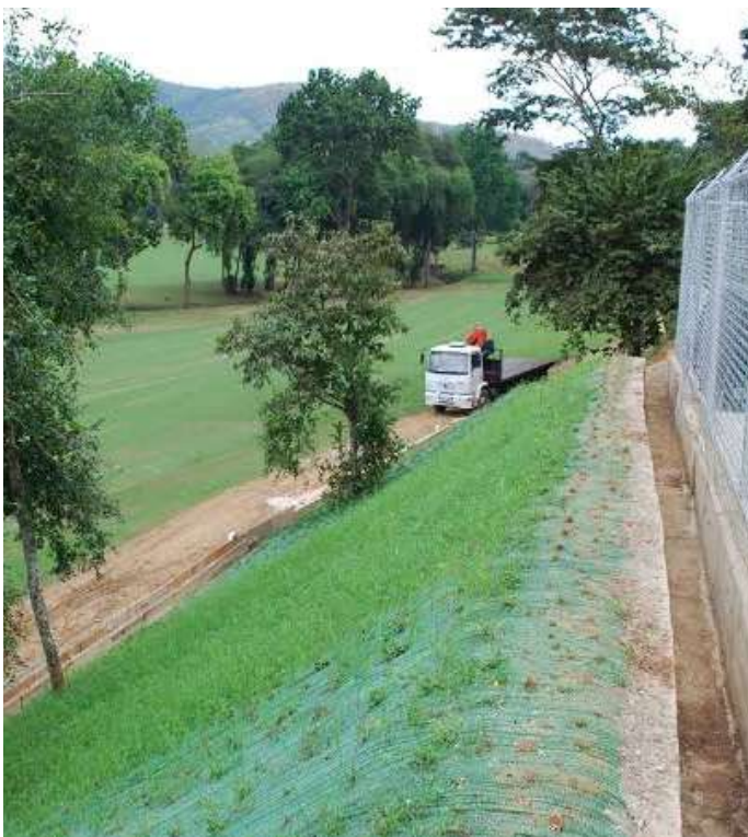
Slope Protection with Geomat
