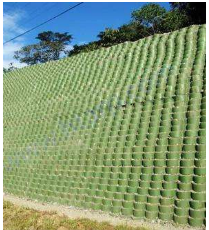
Retaining wall with Geo Cell
