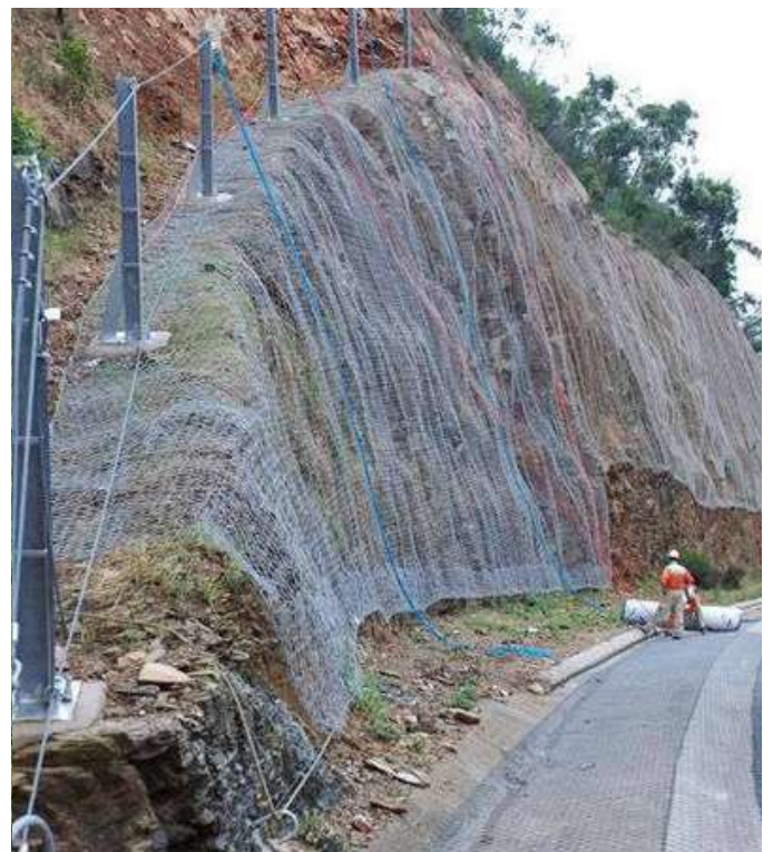
Rock fall Netting work
