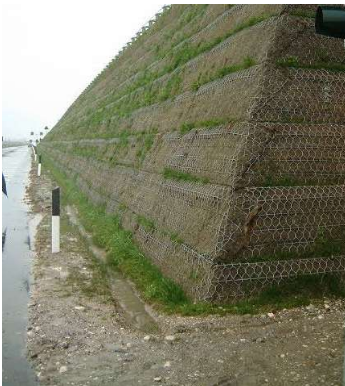
Retaining wall with Green Facia
