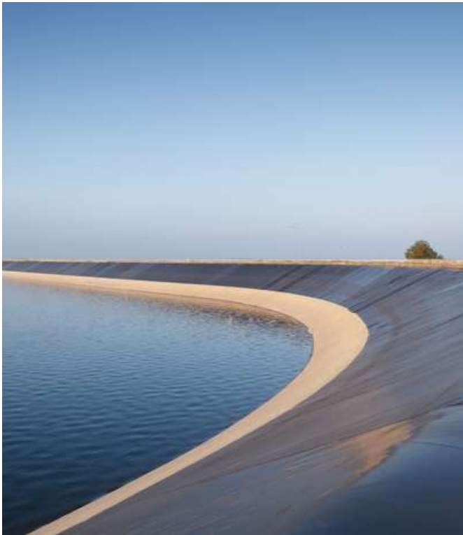
Canal Lining with Geomembrane
