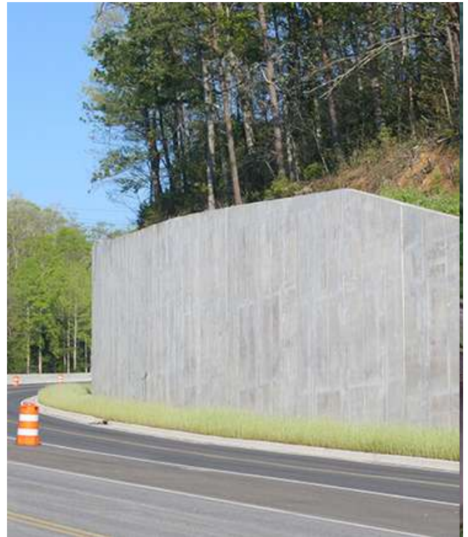
Construction of RCC Retaining walls
