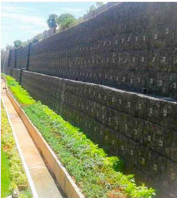
Soil Nailing Work
