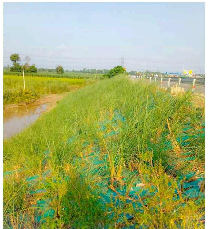
Slope Protection with Geogreen Blanket
