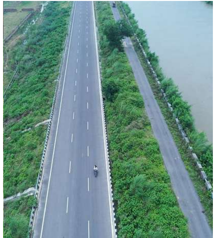
Slope Protection with Coirmat
