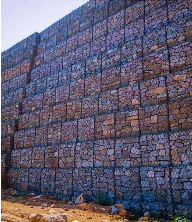
Gabion Gravity Retaining Wall
