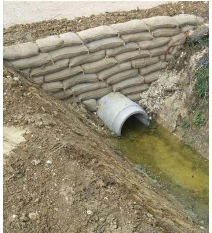
Culvert Protection with Geo Textile
