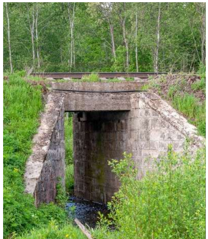
RCC Box Culverts
