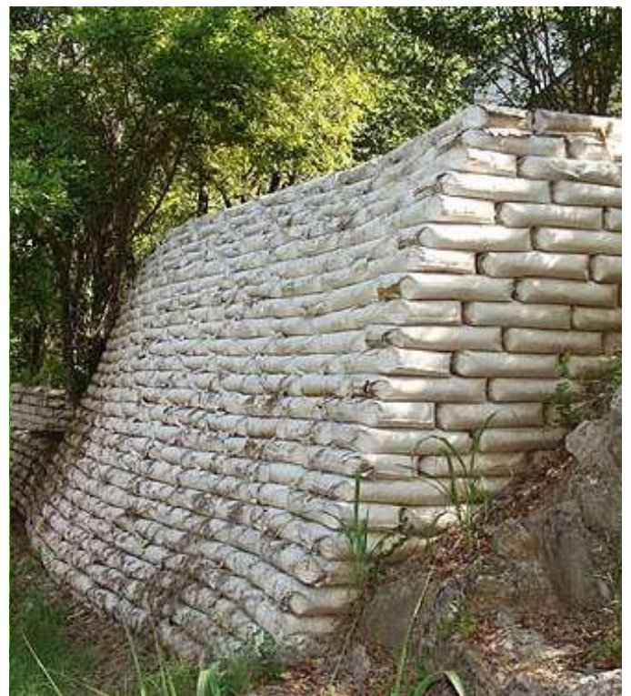
Retaining wall with Geo Textiles
