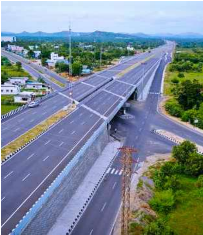
Construction of ROB/VUP
