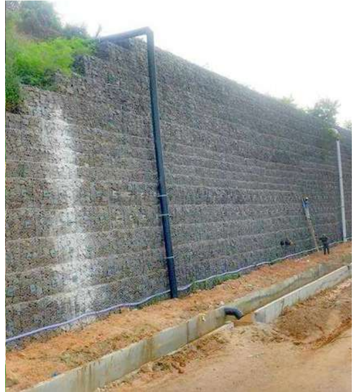
Gabion wall with Geo Grid
