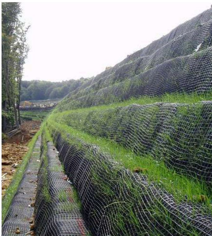
Retaining wall with Geo Grids
